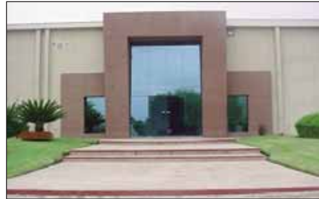
Monterrey, Mexico Manufacturing and Distribution
